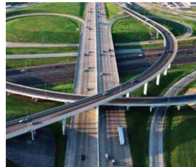
An aerial view of a clover leaf interchange on the U.S. interstate highways.
